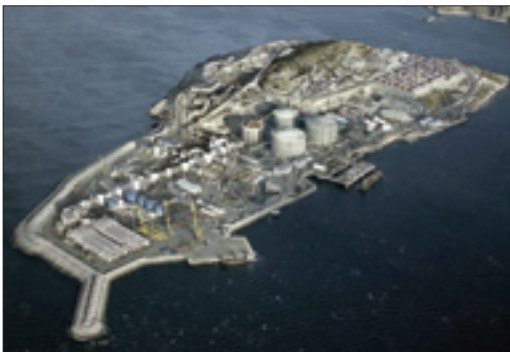
A new gas liquefaction plant in Melkoyja outside Hammerfest in North Norway. Tankers with huge pressure tanks are used to transport the gas.
