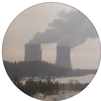
Most new nuclear plants have become safer, but if accidents occur they can be catastrophic. Little CO 2 emissions make them feasible to many countries. The picture shows vapor coming out of cooling towers.
