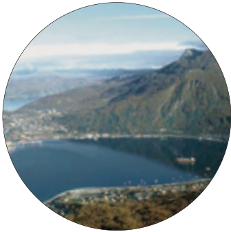
Narvik in northern Norway is going to the main Atlantic port of the N.E.W. Siberian railway system.
