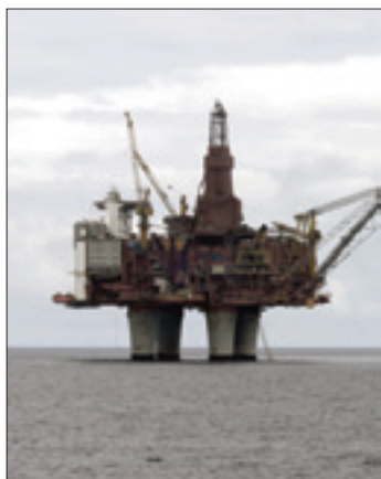
To be able to drill for oil out in the sea opened up huge areas for oil and gas extraction.
