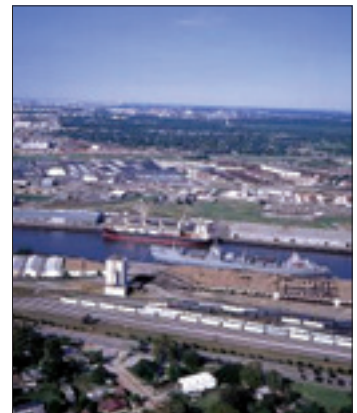
A part of the large depot harbour of Rotterdam. Such harbours are hubs for wider distribution.
