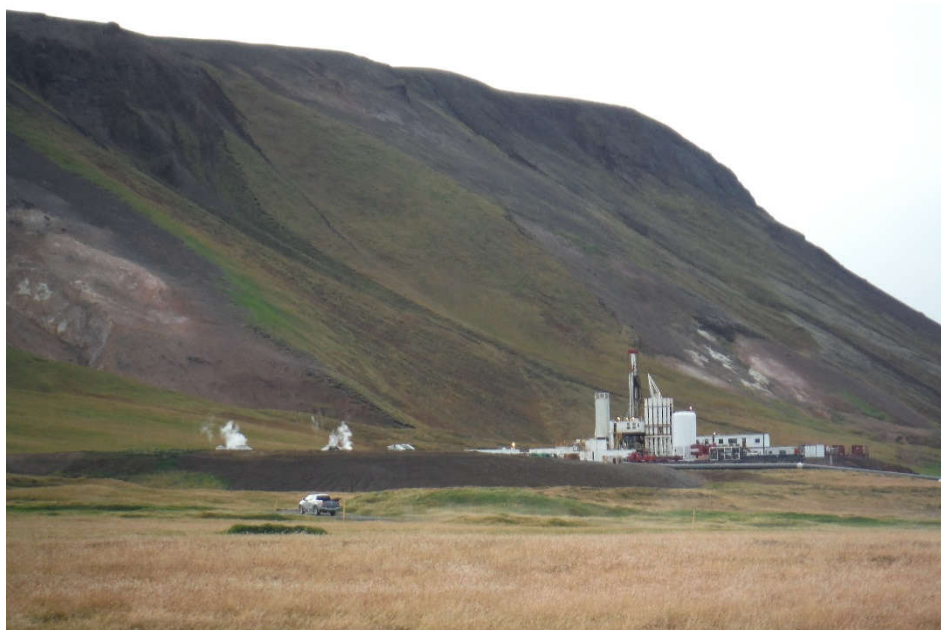
Figure 3: Drilling at Peistareykir.
