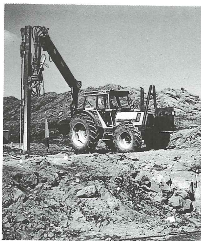
Rock drilling with a hydraulic percussion drill rig designed and assembled in Iceland. (Photo: Birgir Jónsson).
