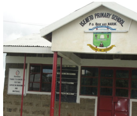
FIGURE 8: Classrooms constructed at Iseneto
