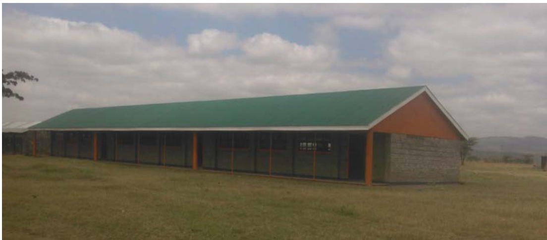
FIGURE 6: New classrooms constructed at Oloirouwa primary school
