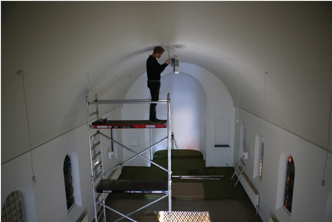
Installation of Inlight. Photo Kolbrún Vaka Helgadóttir.
