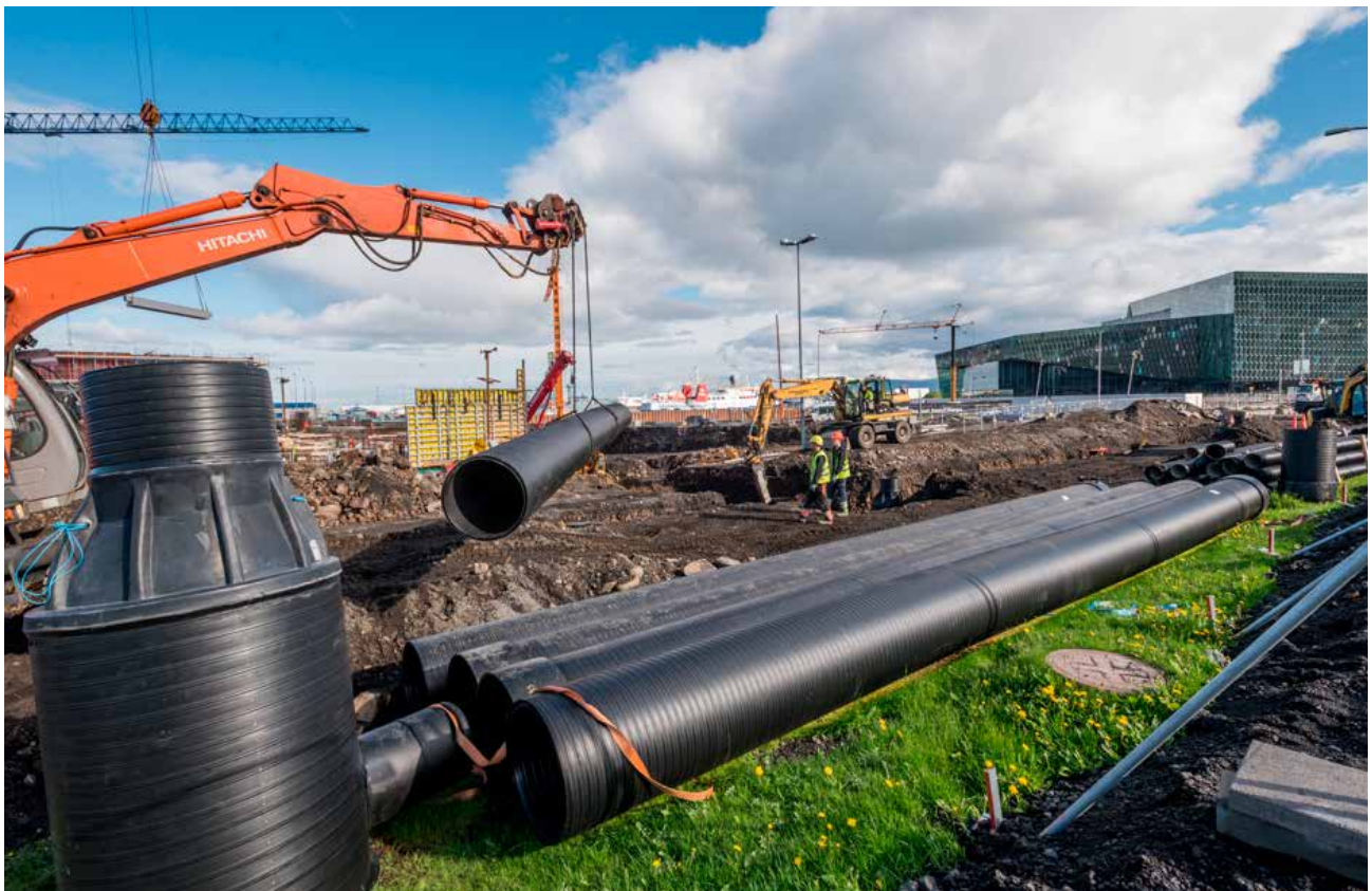
Construction in central Reykjavik. Weholite pipes in the foreground.
