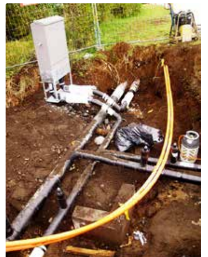
New connections, valves and custom-built pump made by Set Pipes.
