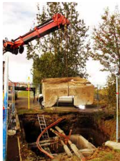
Earlier, the upper part of the well had been lifted from the ground.
