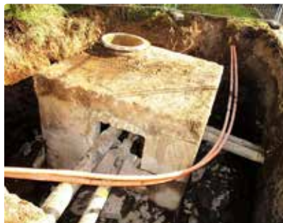
Cleared from the well and it sawn apart horizontally.
