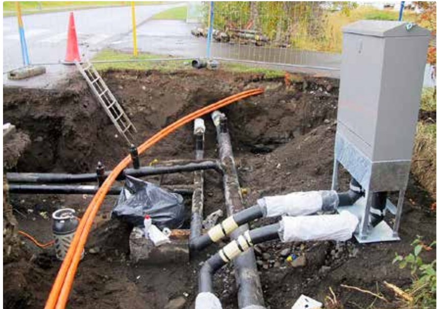
These pictures were taken when the concrete well was removed from Vestursíða in Akureyri, Iceland. The custom made pipes were designed and produced by Set Pipes.
