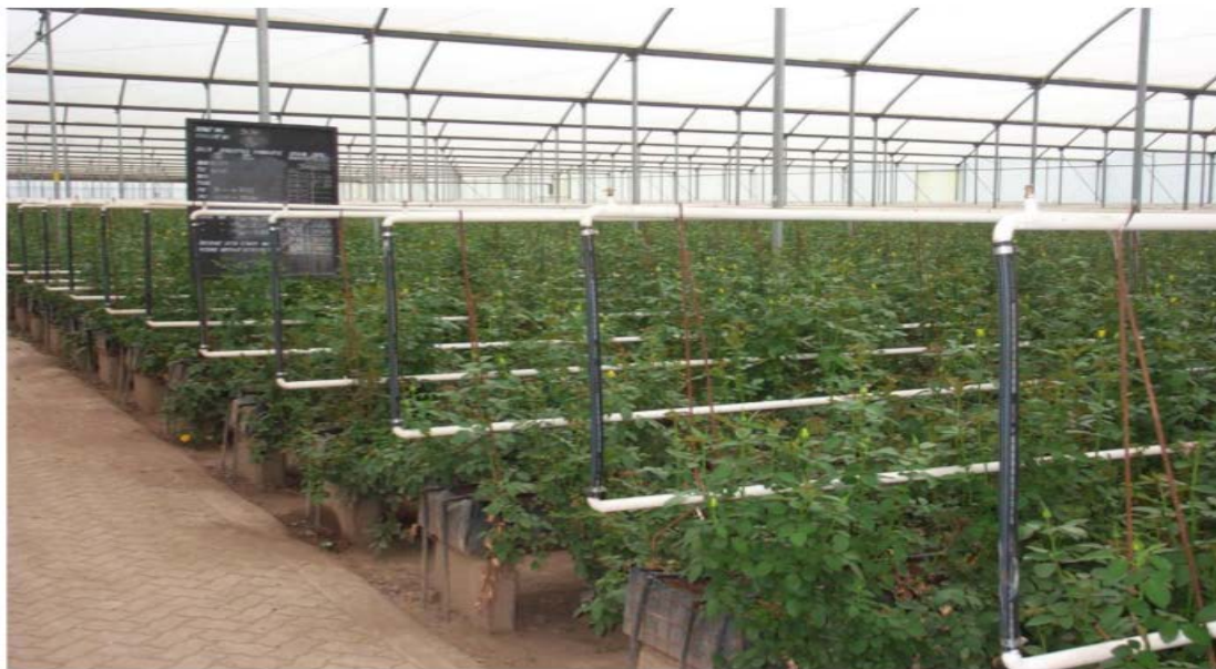
FIGURE 6: Oserian greenhouse heating using geothermal
