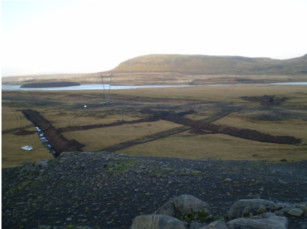
Figure 2. Overview of the powerhouse area. Trenches 1-4 already excavated
