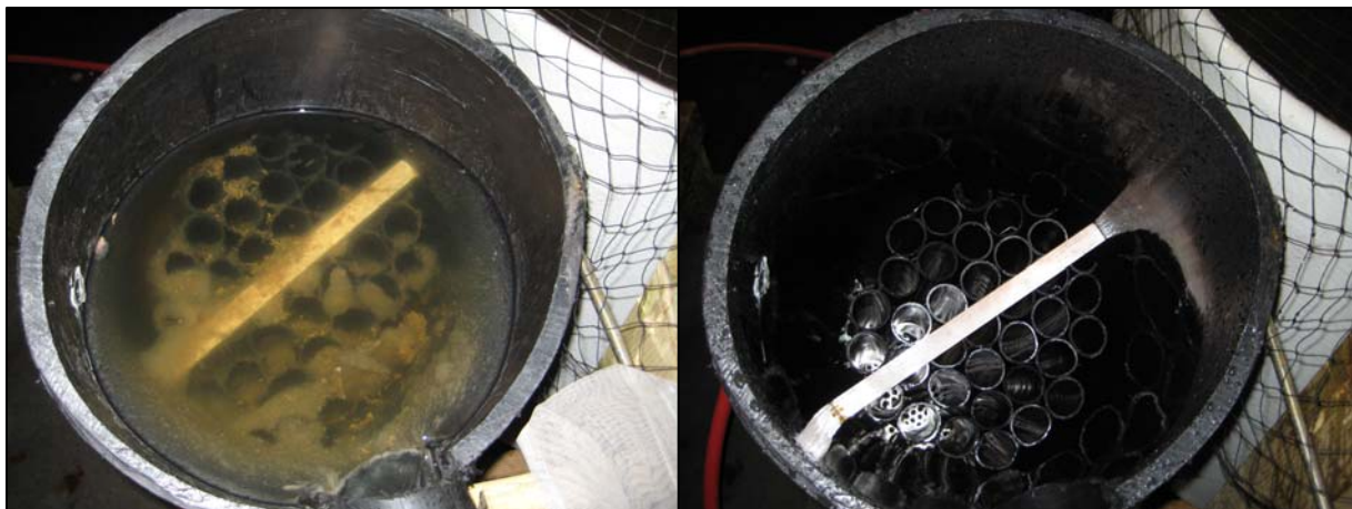
Figure 3.1 Tube settler before and after back flushing
