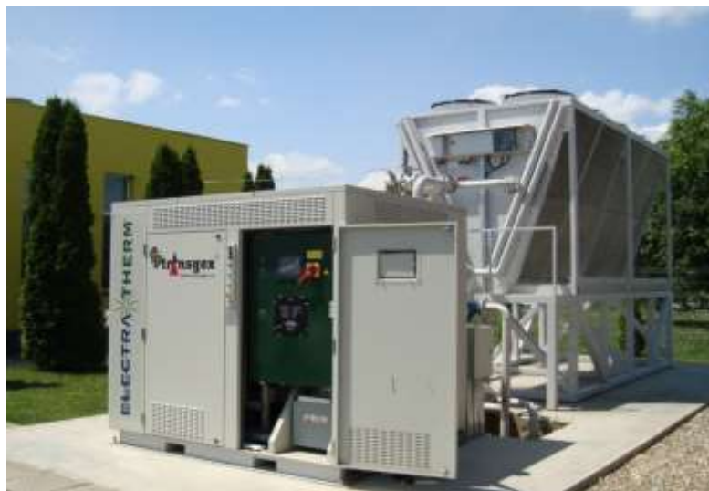
50 kWe Binary Cycle ORC Geothermal Power Plant installed in Oradea by Transgex Company
