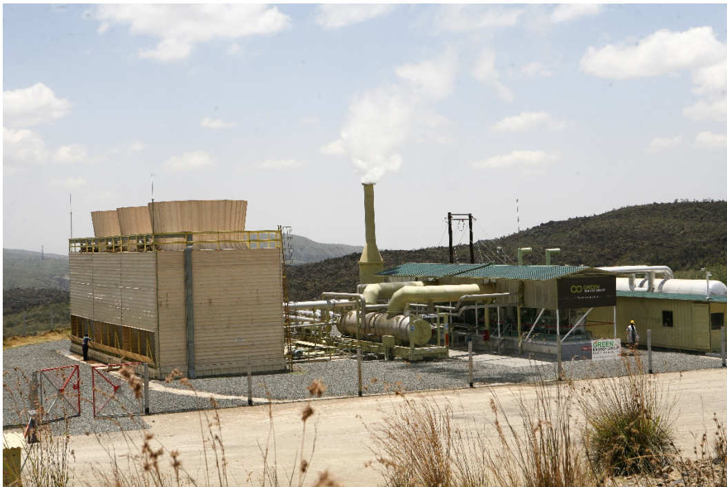
FIGURE 3: A 5 MW well-head at Olkaria geothermal field
