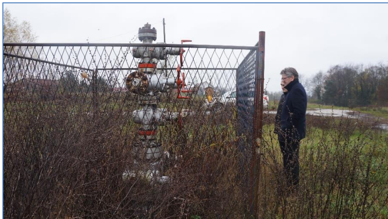
Figure 8.1. Geothermal well in Križevci
