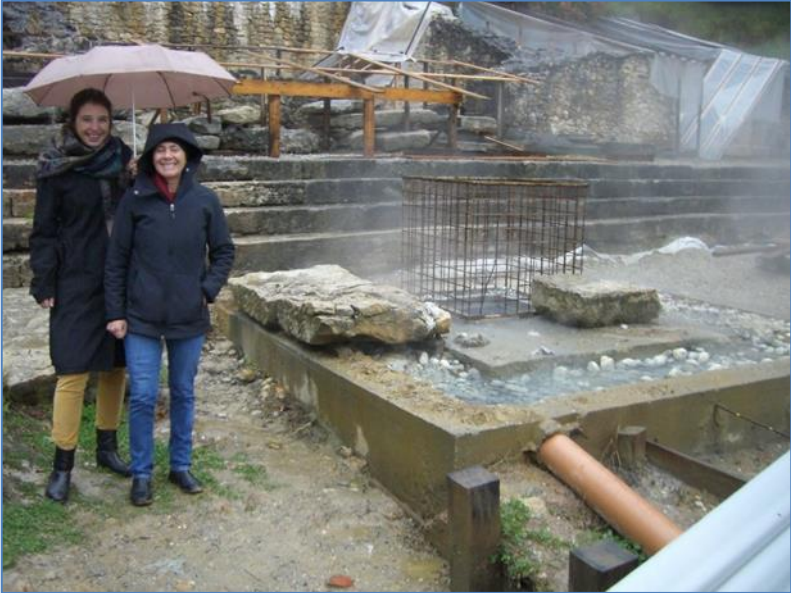
Figure 9.2. Artesian well in Varaždinske Toplice
