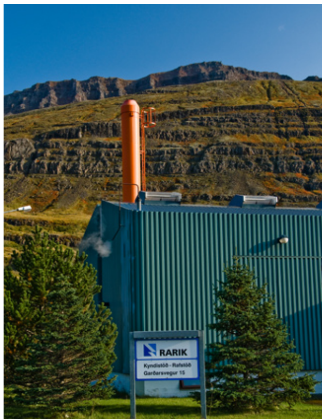
Seyðisfjörður District Heating Plant
