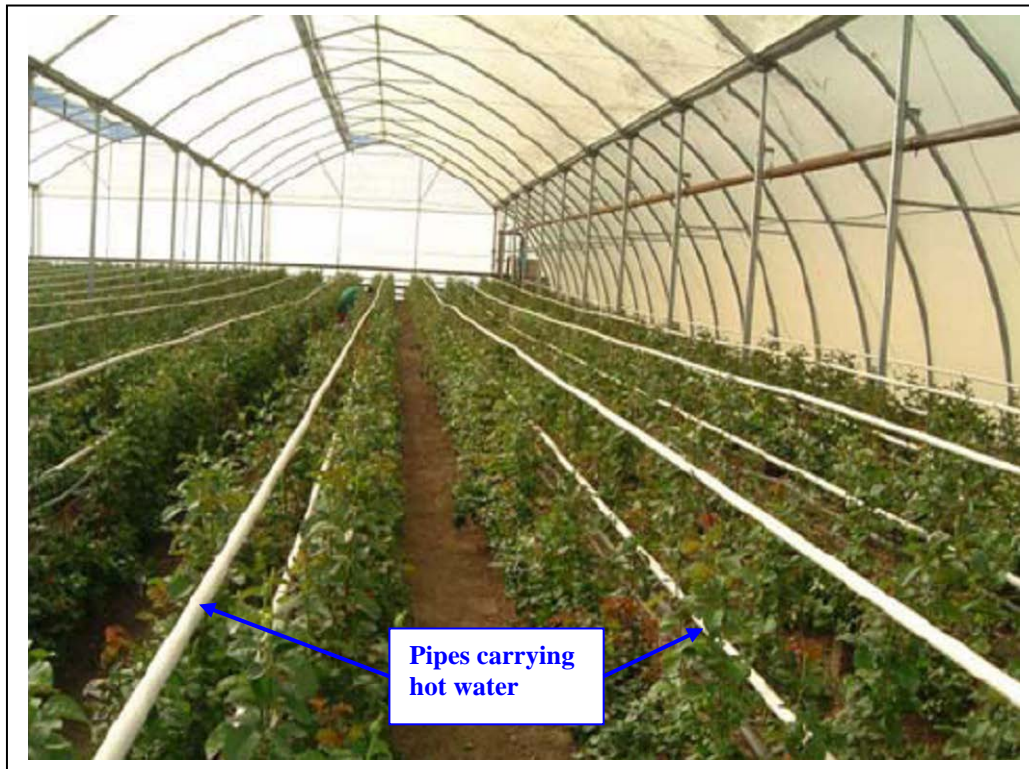
FIGURE 6: Geothermal greenhouse heating at Oserian Company, Kenya
