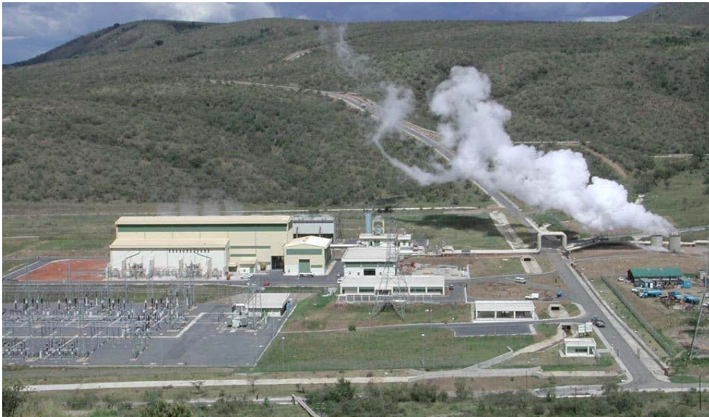
FIGURE 5: Olkaria II power station, commissioned in 2003
