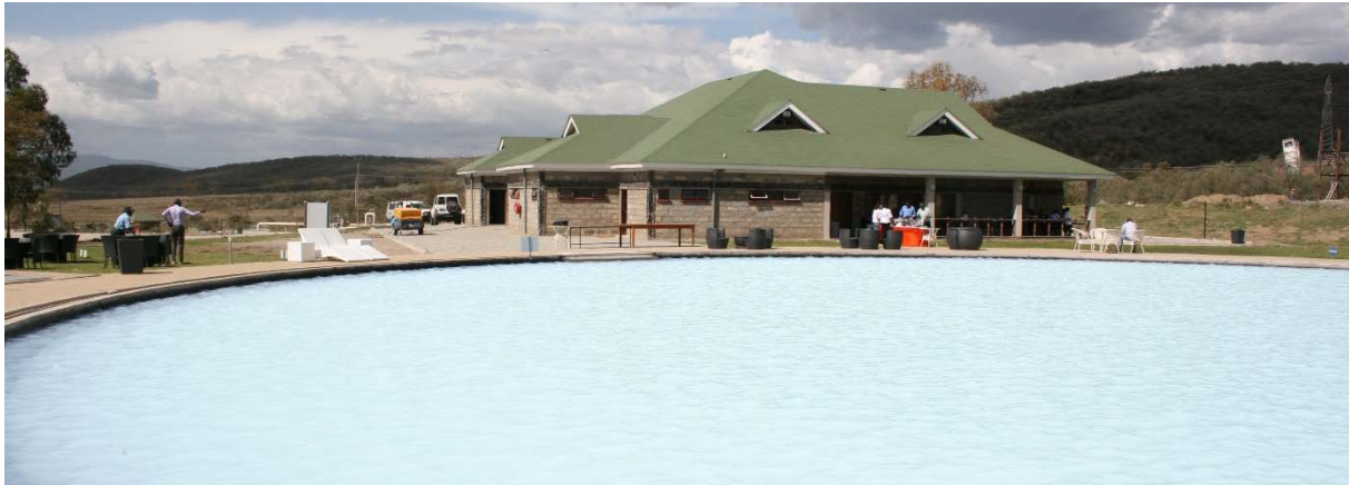
FIGURE 5: The new geothermal spa in Olkaria, Kenya
