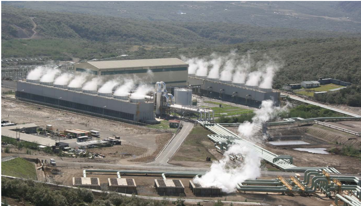
FIGURE 3: The new Olkaria IV power station in Kenya, opened in mid 2014, with an installed capacity of 140 MWe from 2 turbines
