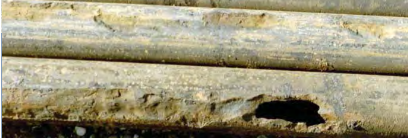
Example from Nagra Borehole Weiach:- Longterm monitoring system
