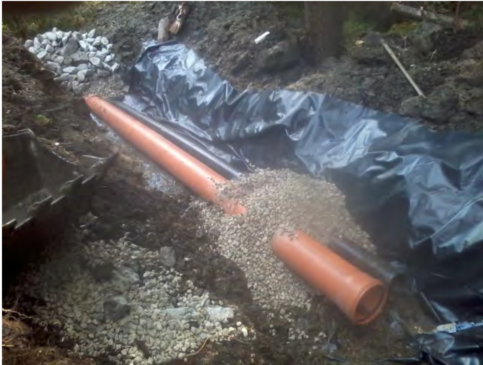
Figure 12. Drainage pipe, discharge pipe, proofing, gravel.
