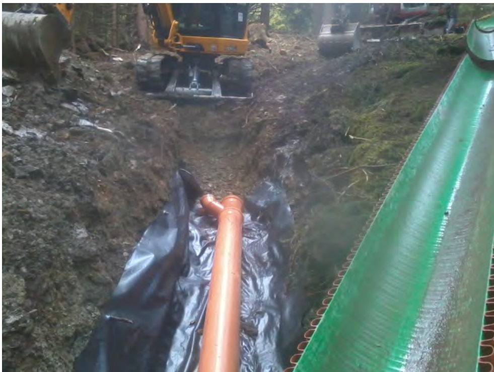
Figure 13. Half-shell parts of drainage pipes.
