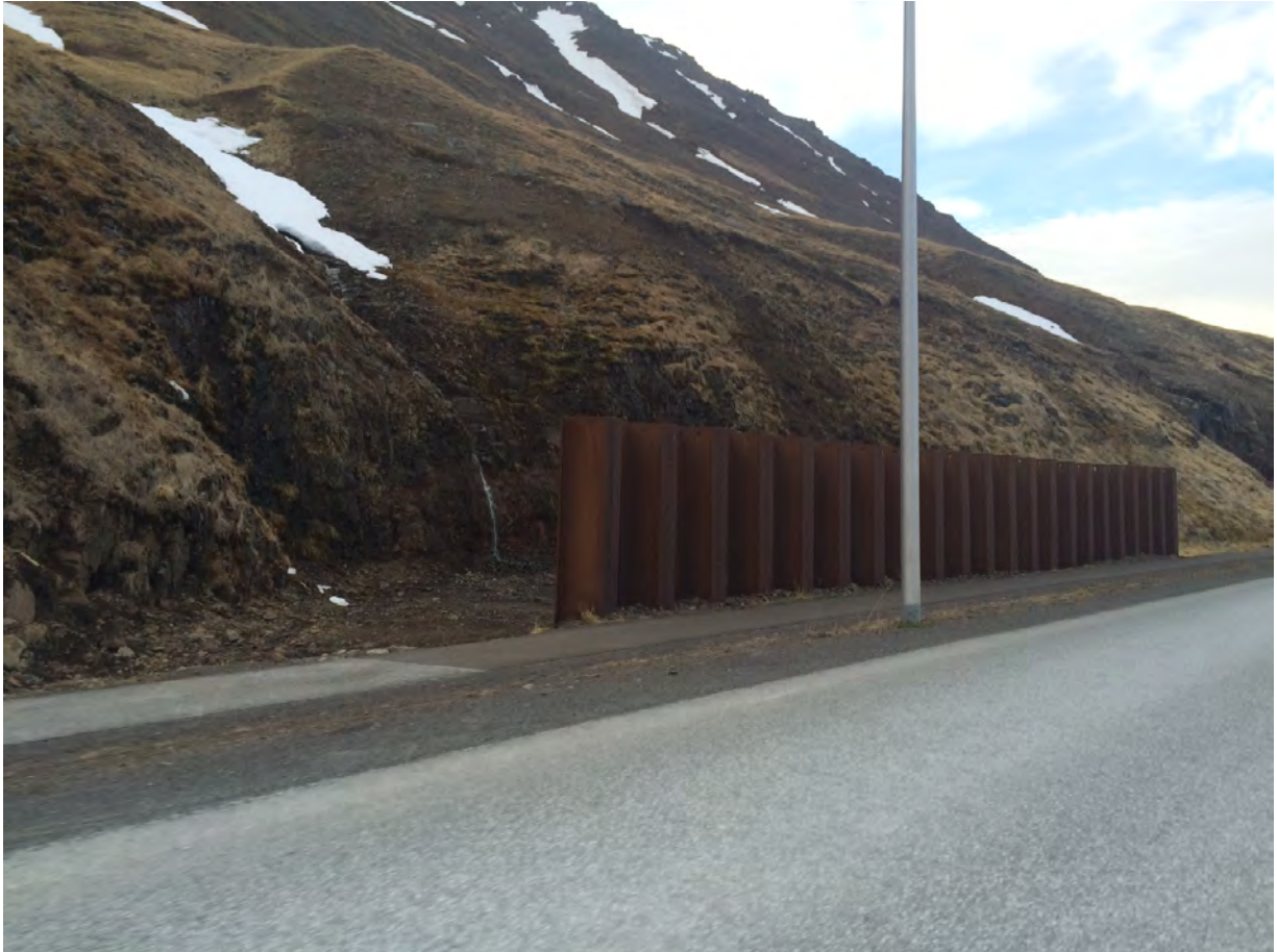
Figure 25. A steel wall above the road below Eyrarhlíð in NW-Iceland for reducing the frequency of snow avalanches reaching the road. Photograph: Jón Kristinn Helgason.
