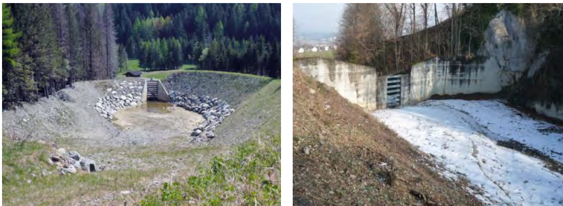
Figure 18. Bed-load samplers in Switzerland made of fill material (left) and concrete (right) with a by-pass structure made of concrete and steel bars (Margreth, 2015). The steel bars separate water from the bed-load. Such structures are often built in Alpine countries. Photographs: Stefan Margreth.
