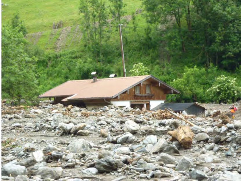
Figure 9. A building hit by a thick debris flow on 8 June 2015 in the village of Sellrain, Tyrol, Austria. Photograph FTD, 2015.
