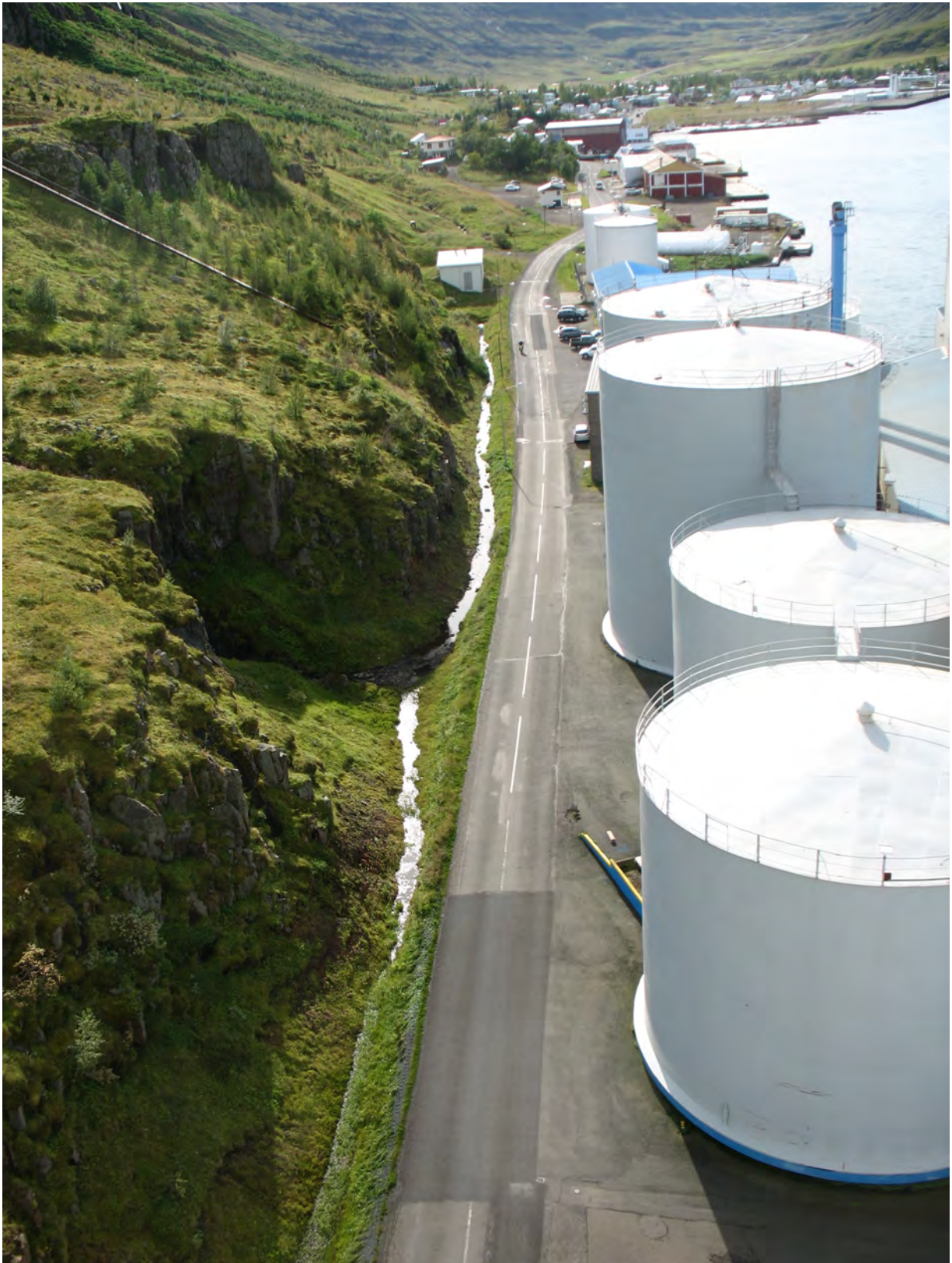
Figure 24. The main tanks of the SR fish factory below Pófi where point protection by a concrete wall might improve the safety.
