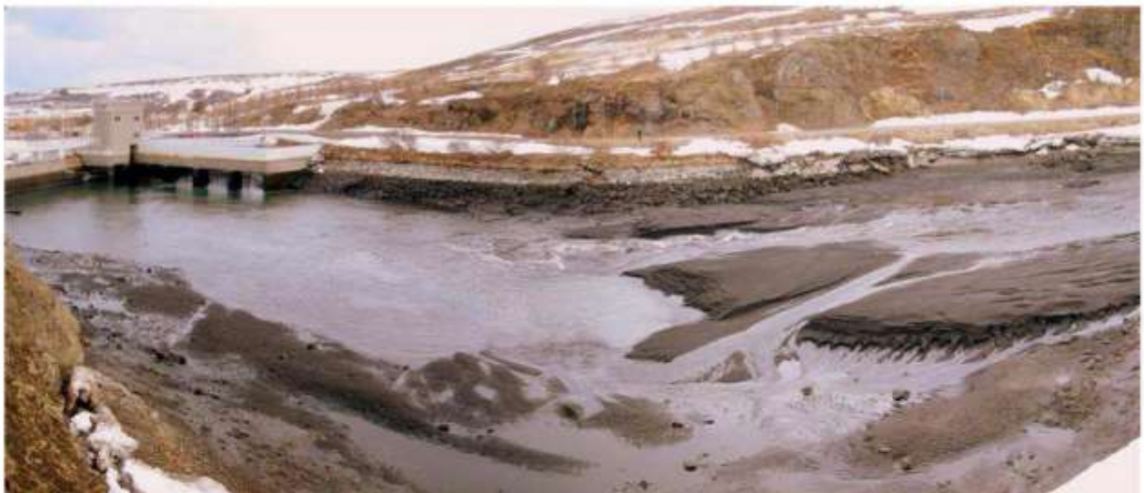
Figure 5 – Laxá II intake pond during flushing.
