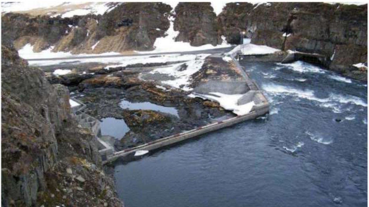
Figure 8 – intake pond at Laxá III during flushing. The intake can be seen on the right.
