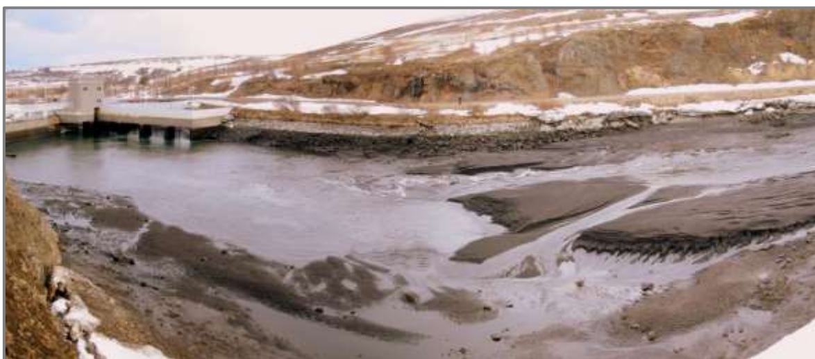
Figure 13: Laxá II head-pond during draw-down and flushing (Ref. 3)
