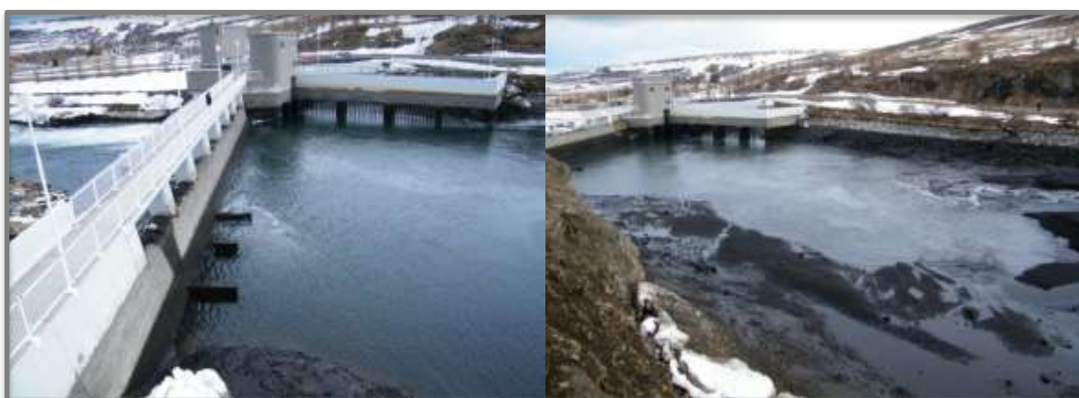
Figure 11: Laxá II Dam and Intake to Laxá 2 Hydropower Plant (Ref. 3)
