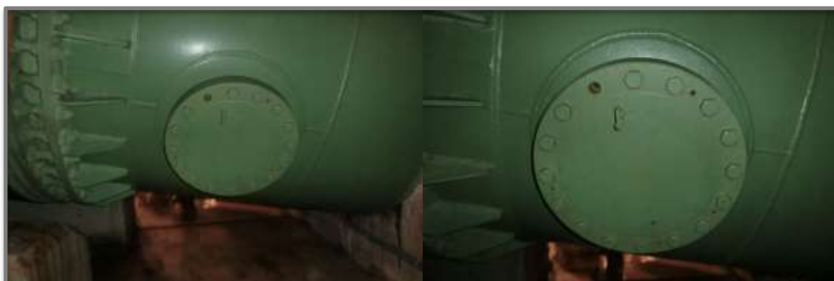
Figure 31: Location for installation of a SMOOTH sediment sampler for manual and automatic sediment measurements
