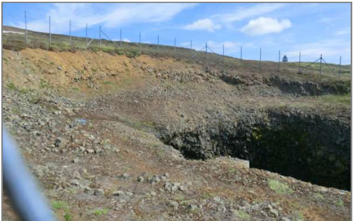
Figure 25: Surge shaft opening as it is today
