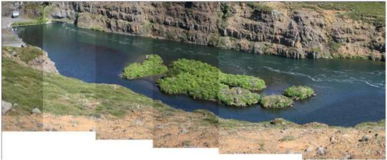
Figure 6 – top view of the Laxá III intake pond. Almost all the discharge flows by the far bank. Accumulation of sand can clearly be seen at stabilized operating conditions.
