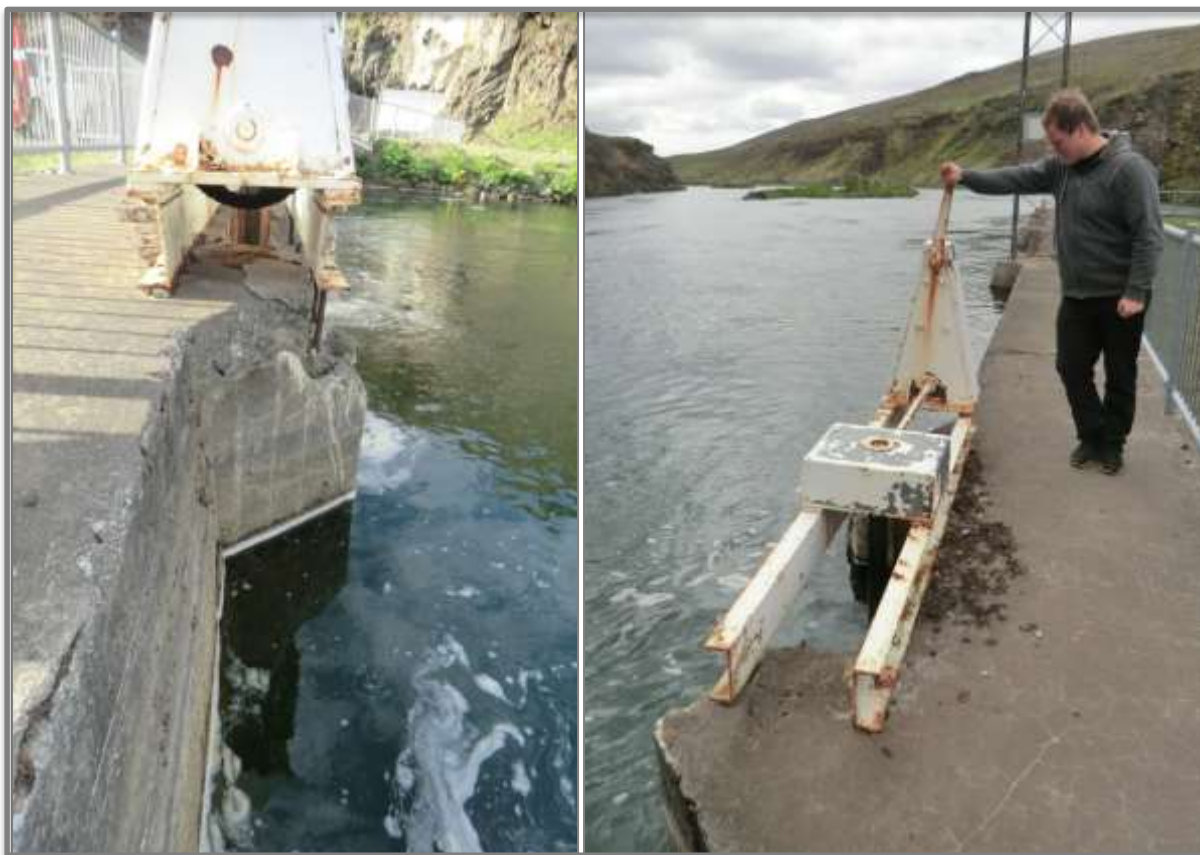
Figure 10: Hoisting arrangement for the bottom outlet gate, possible sediment flushing gate?
