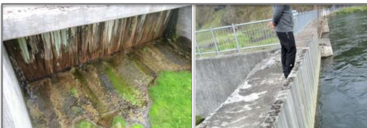
Figure 8: Bay with vertical stop-logs upstream of concreted bays with downstream embankment
