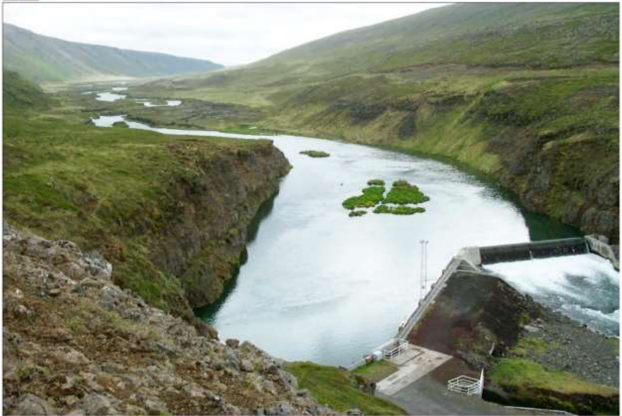
Figure 7 – overview of the intake pond at Laxá III. 80% of the flow through the pond is by the left bank. This is the location of the original main river bed.
