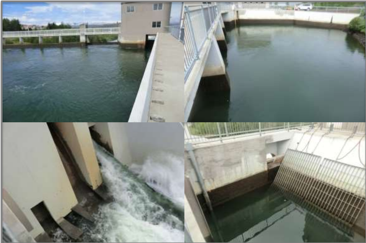
Figure 15: Dam, intake bay with "skirt-wall" and water and ice passage arrangements at Laxá II Dam
