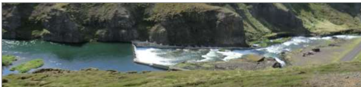
Figure 7: Left side of the dam with free overflow spillway and the existing bay with vertical stop logs, seen from the right bank
