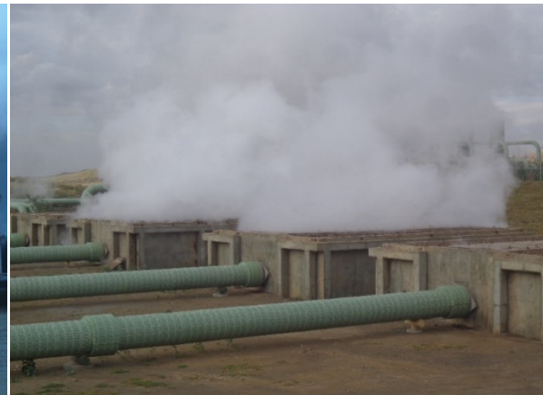
FIGURE 11: Olkaria IV steam venting station
