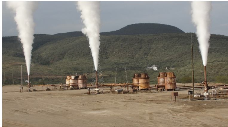
FIGURE 7: Olkaria well-915 pad with three wells
