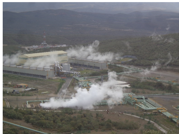
FIGURE 6: Olkaria IV power plant
