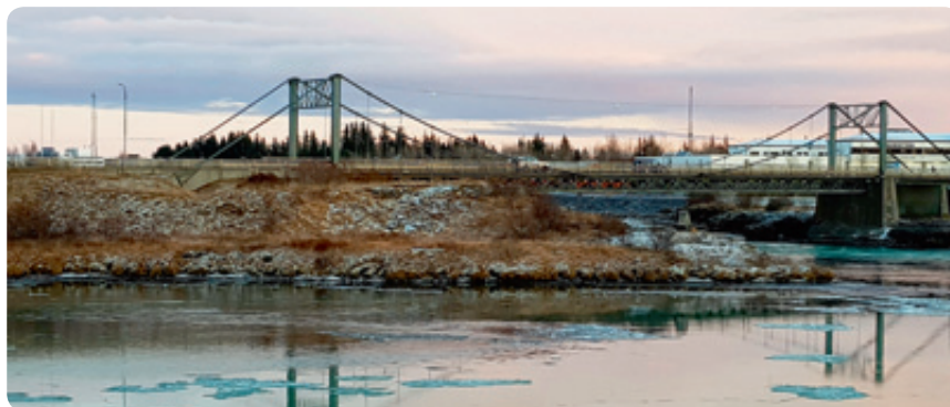
A suspension bridge over Ölfusá River was built in 1945. The bridge is 84 meters long and is in the town Selfoss.
