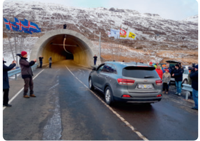
Last year a 7.9 km (4.9 mi) long tunnel, named Norðfjarðargöng, were opened between Neskaupstaður and Eskifjörður.
