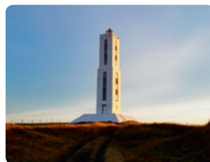
Built in 1938-1939, the Knarrarósviti lighthouse was the first one in Iceland to be built out of reinforced concrete.
