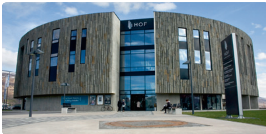
Hof is a cultural building designed for music and other performing arts, as well as top-notch facilities for conferences and meetings, receptions, parties and exhibitions.
