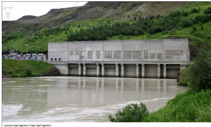
Picture 4: Búrfell Hydropower Station in Þjórsá, southern Iceland. Photo: Ásgeir Eggertsson/Landsvirkjun
