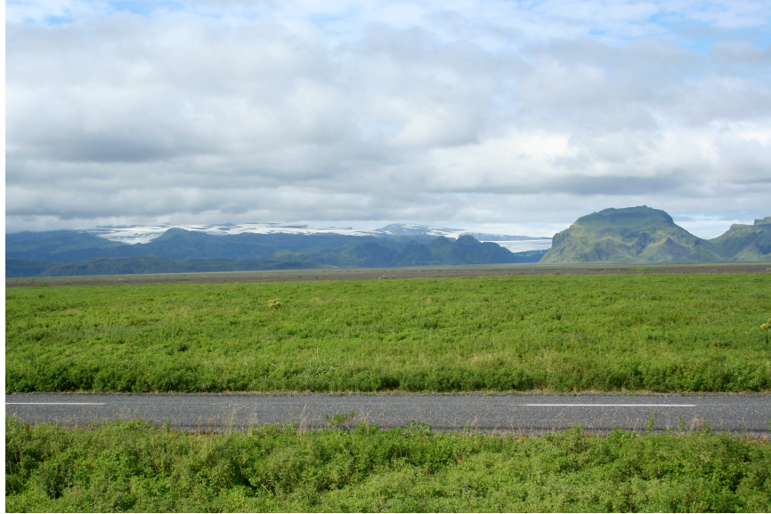
Picture 9: The road over Mýrdalssandur crosses a flood plain, which is the likeliest runway of melt water during eruptions in the volcano Katla. Such melt water floods can cause heavy damage to roads (Björnsson et al., 2011). Photo: ÁJ
