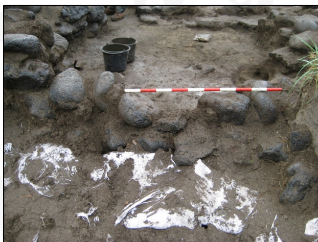
Figure 7 West wall of the room. White sandbags in front to keep the wall in place as it is on the erosionline.
