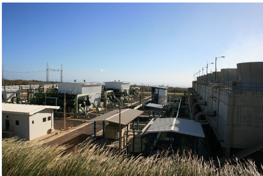
FIGURE 2: The Las Pailas binary geothermal power plant in Costa Rica
