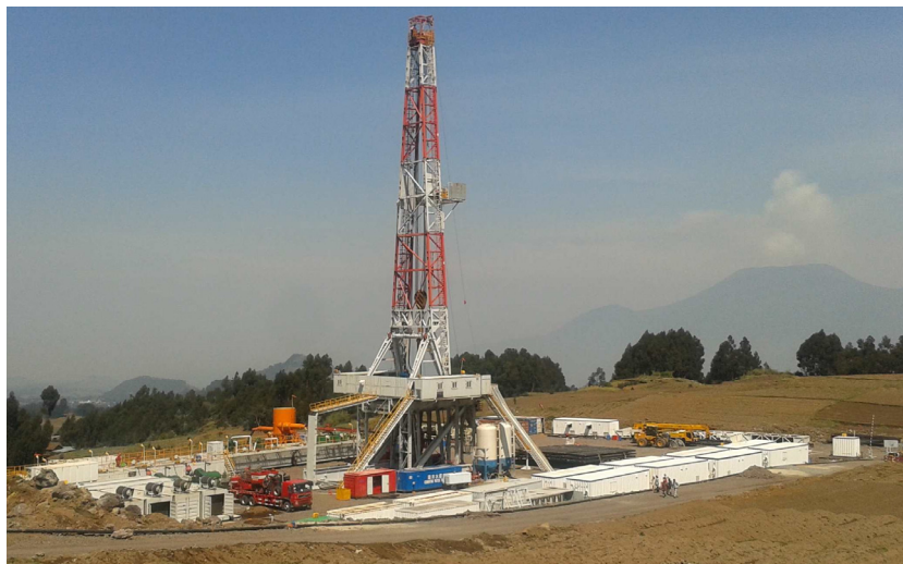
FIGURE 6: Karisimbi geothermal exploration drilling project, July 2013
