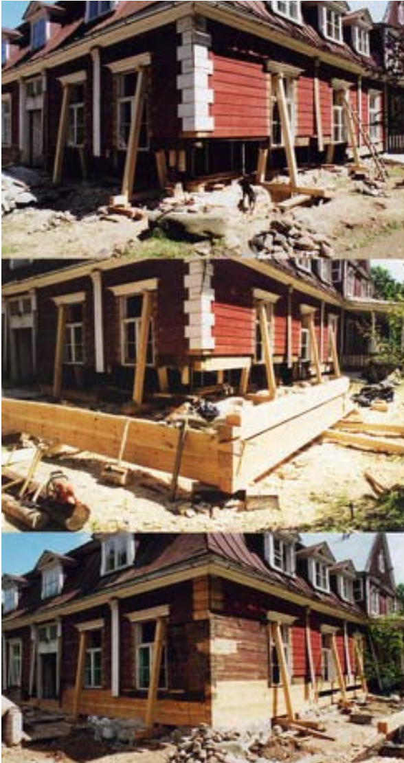
Ungurmuiza Manor in Latvia after restoration. Damaged timber sections have been changed. The roof is covered with new shingles, painted with a mixture of Estonian wood tar and Swedish red paint. Photo: Ilmars Dirveiks.
