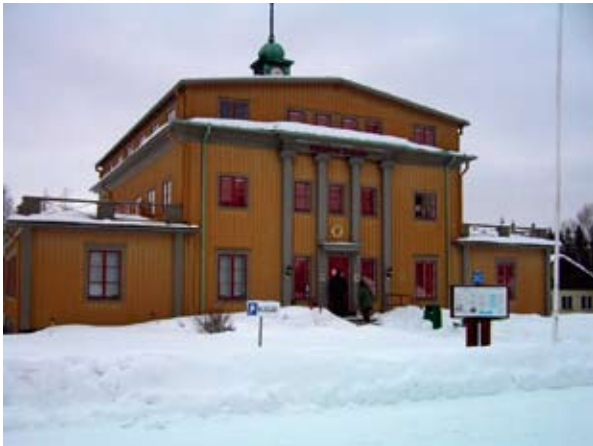
Berggrum Boliden museum is situated in the Boliden mining company's former director's villa. Photo: Torkel Molin.
