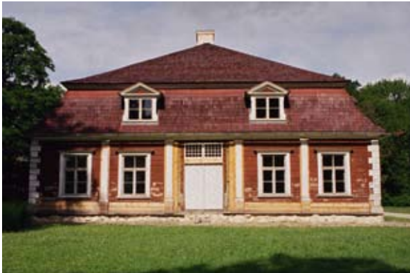
View of the south facade of the Ungurmuiza manor after restoration. Roof shingles are painted with red colour tar. Photo by Ilmars Dirveiks.
