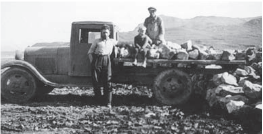
Photo 6.24 Gathering stone to construct a levee to stop flooding in 1940
