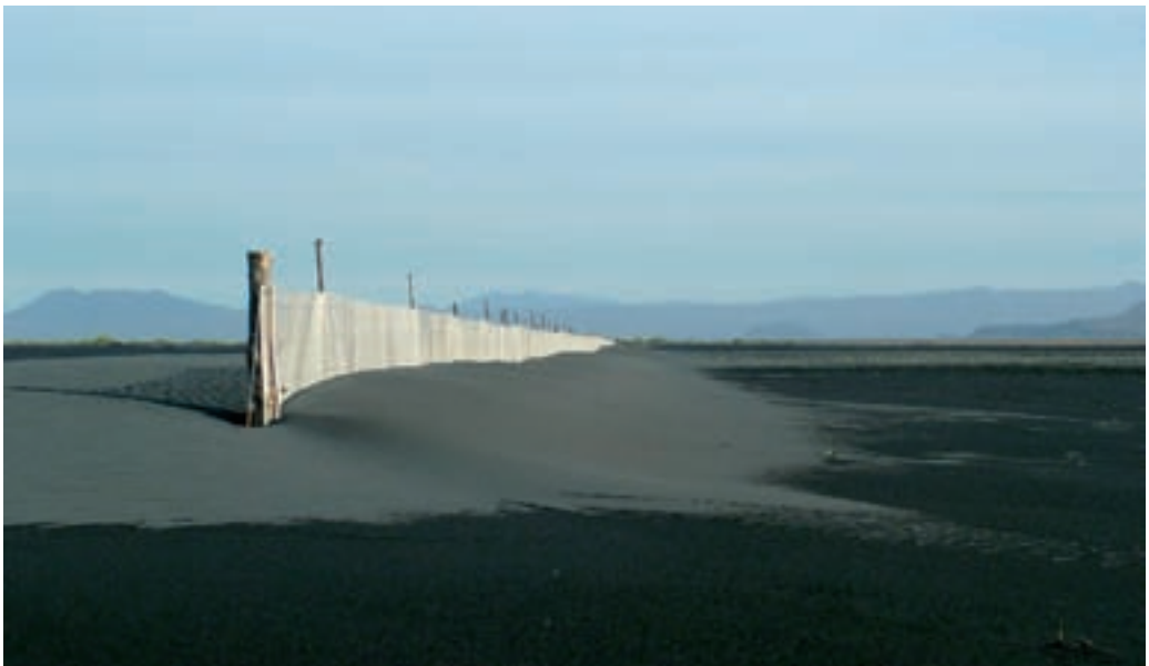
Photo 6.19 New style of timber and wire fence tested for efficiency
