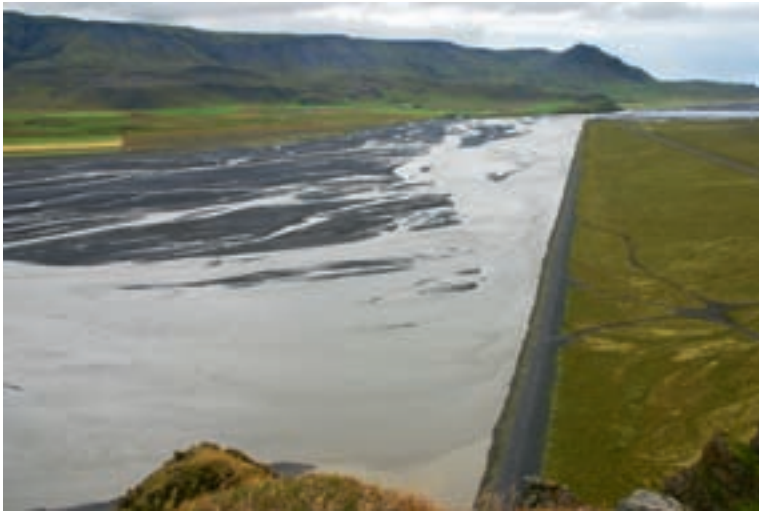
Photo 6.25 Levees to control river channels and to reduce flooding and consequent land loss
