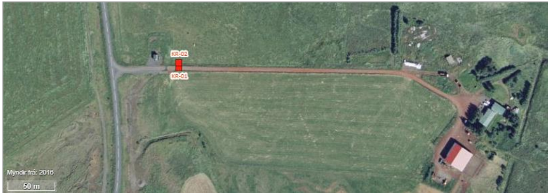
Figure 114. Overview of the production wells in the Kringla well field (NEA's Geoportal).
