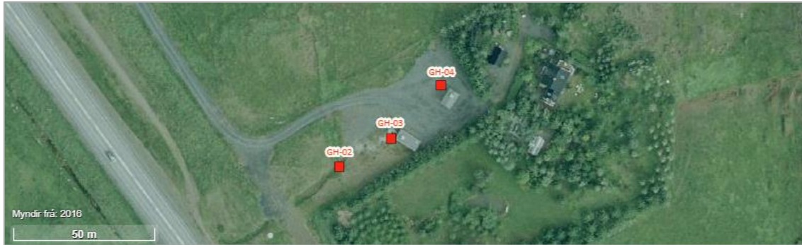
Figure 126. Overview of the production wells in the Gljúfurárholt well field of the Hveragerði geothermal field (NEA's Geoportal).
