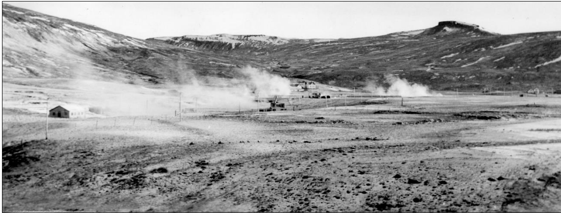
Figure 17. The steaming Suður-Reykir subfield due to runoff from the free-flow wells before they were harnessed. (Photo archive: Orkuveita Reykjavíkur, 2018).
