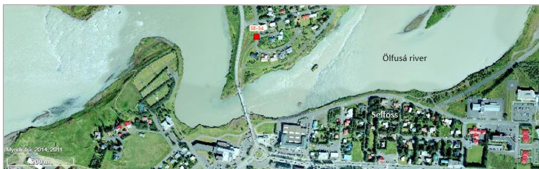
Figure 121. Overview of the production well SE-34 in the Jórutún well field of the Selfoss geothermal field (NEA's Geoportal).
