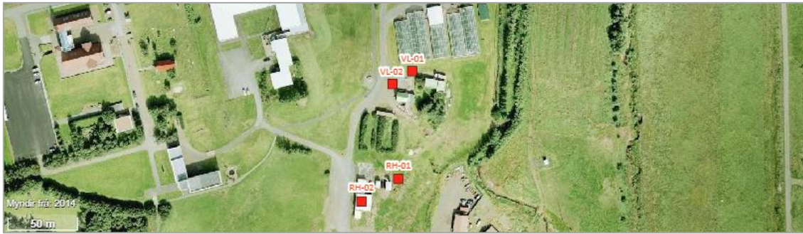
Figure 35. Overview of the production wells in the Reykholt well field (NEA's Geoportal).
