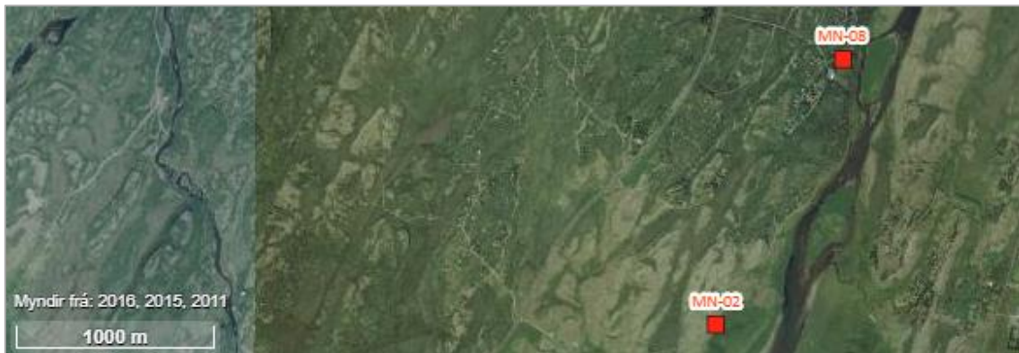
Figure 40. Overview of the production wells in the Munaðarnes well field (NEA's Geoportal).
